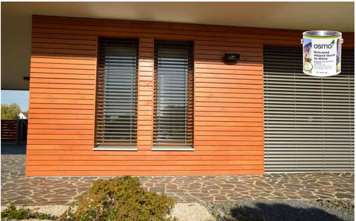
REAL FACADE, Siberian larch, Raute profile 20 x 93 mm, surface treatment OSMO Protective oil stain n. 728 Cedar
