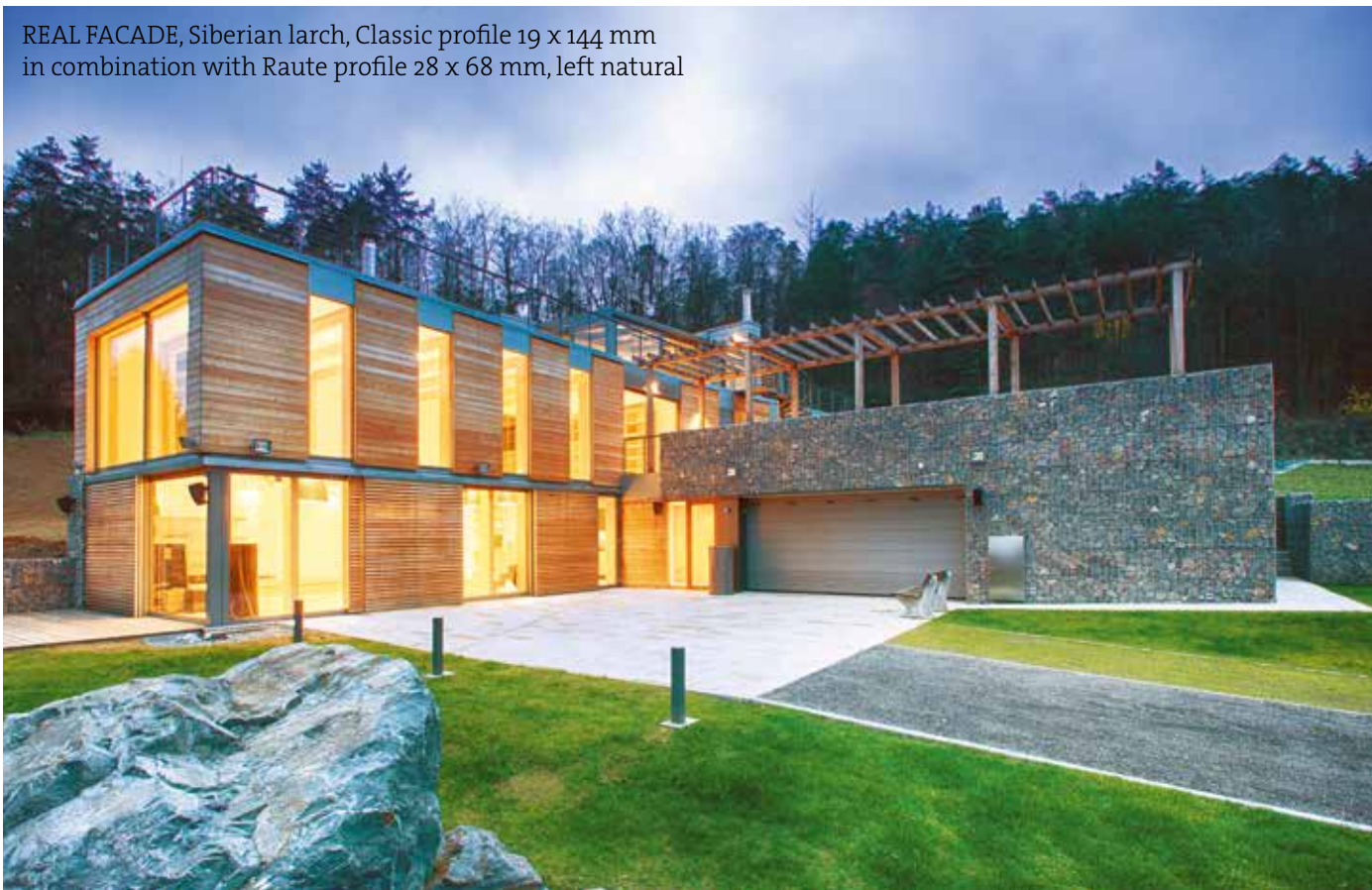
Facade, Siberian larch, planed boards 20 x 95 mm, Surface treatment OSMO Protective oil Extra n. 420 transparent
